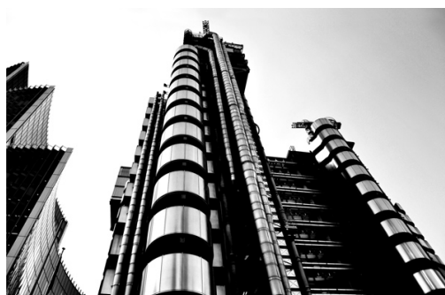
the Lloyd's building
